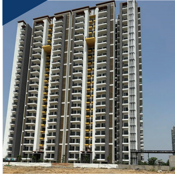
Client Name: County Group Project Name: Coco County
